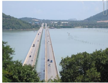
Figure: 3.2 Tinsulanond Bridge Source: http://gotoknow.org/file/krukin/ky4108.JPG
