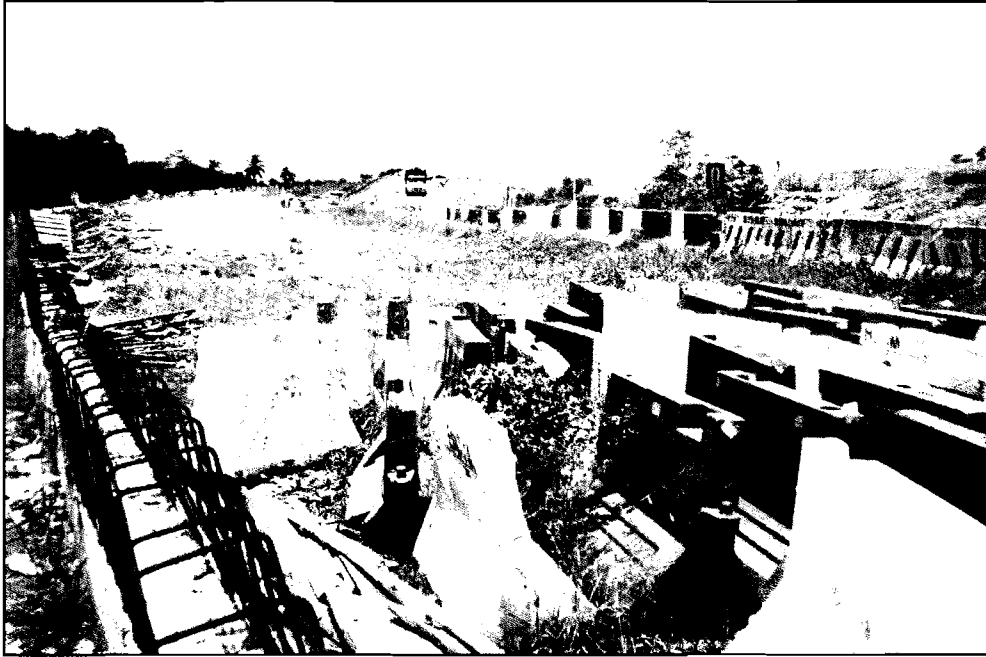
Picture E16: The road construction at Padang Besar
