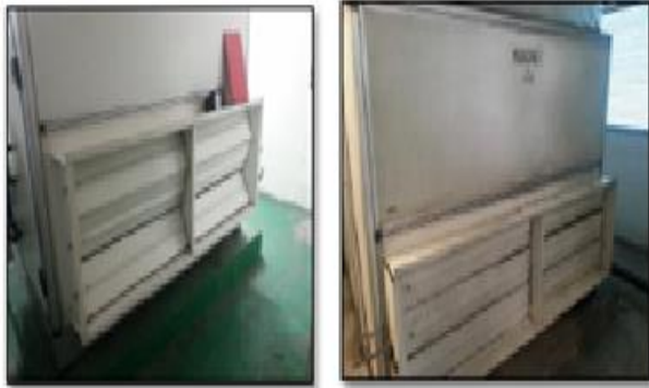
Photo 4 Fresh air dampers in the AHU room were closed
