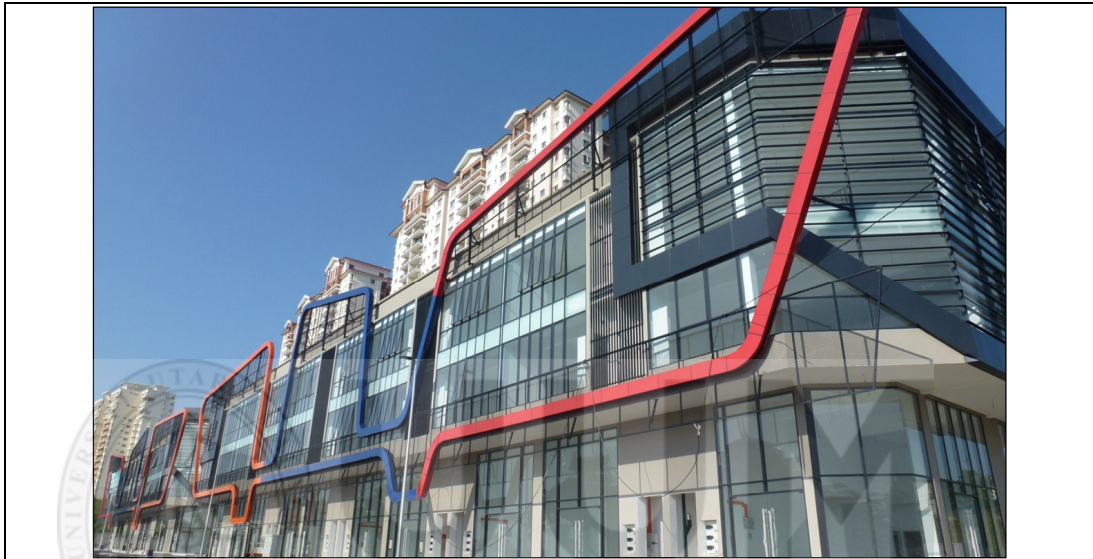
Figure 5.1 Units shop lot, Serdang Perdana, Selangor
