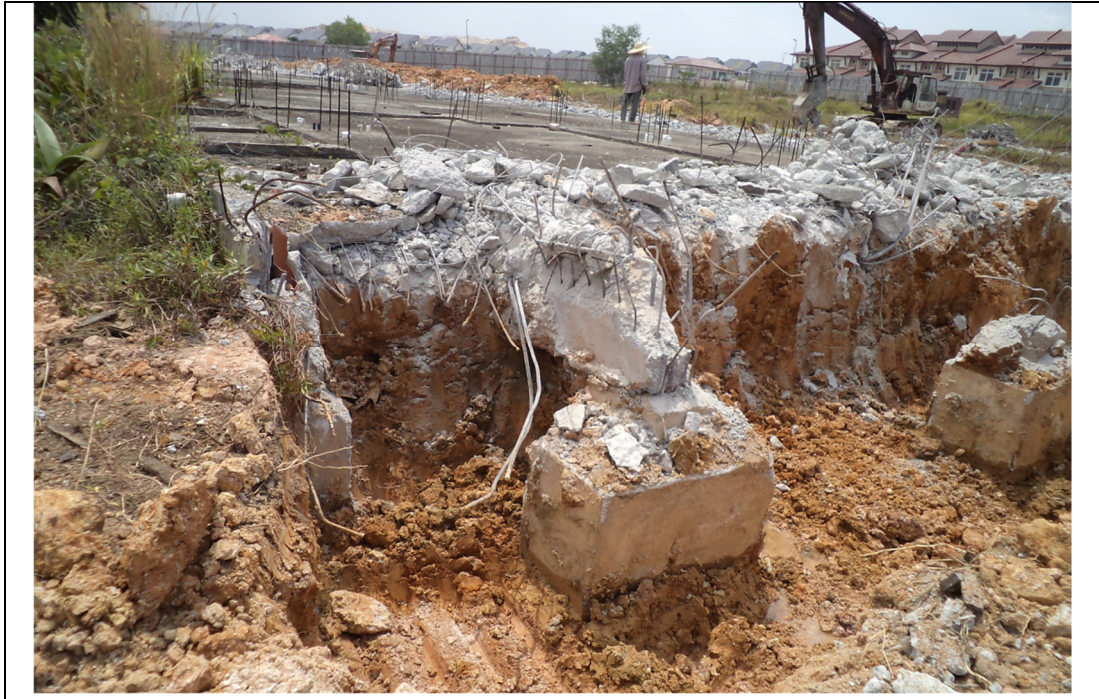
Figure 5.8 Excavation on the ground floor slab.
