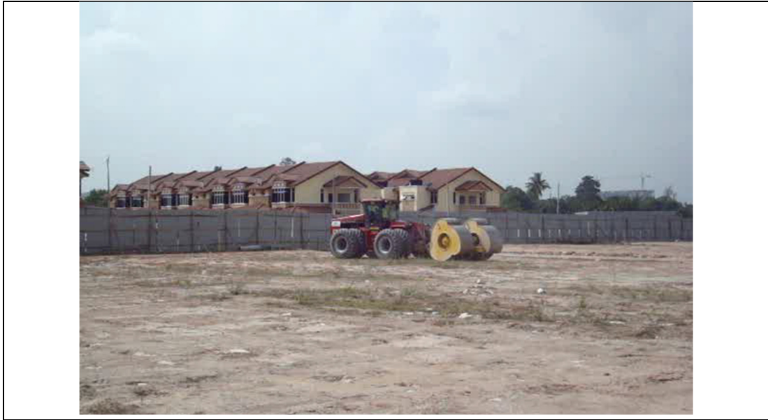
Figure 5.9 Rolling dynamic compaction at the project site
