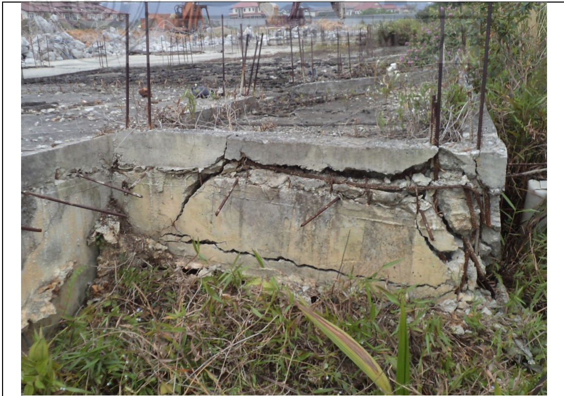
Figure 5.7 Photo of distorted slab and major upheaval.
