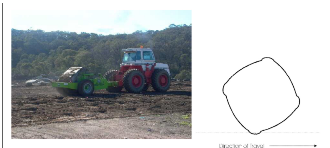
Figure 5.10 Concept of Rolling Dynamic Compaction (Bouazza and Avalue, 2006)
