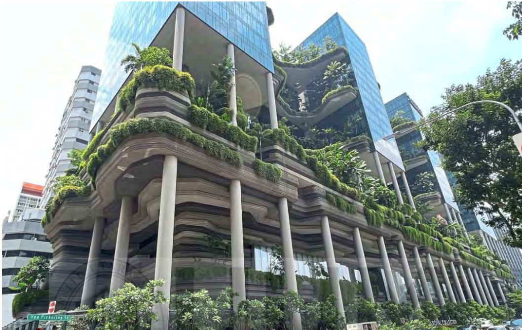
Figure 6-6 Vertical Greenery at Parkroyal Pickering
