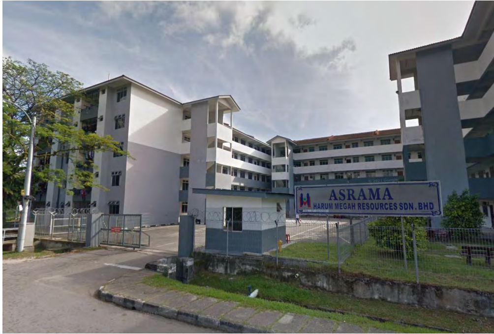
Figure 5-5 Centralise Labour Quarters in Pasir Gudang
