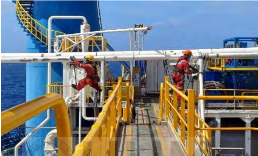
Photo 1: Observation During Working at Height Activity
