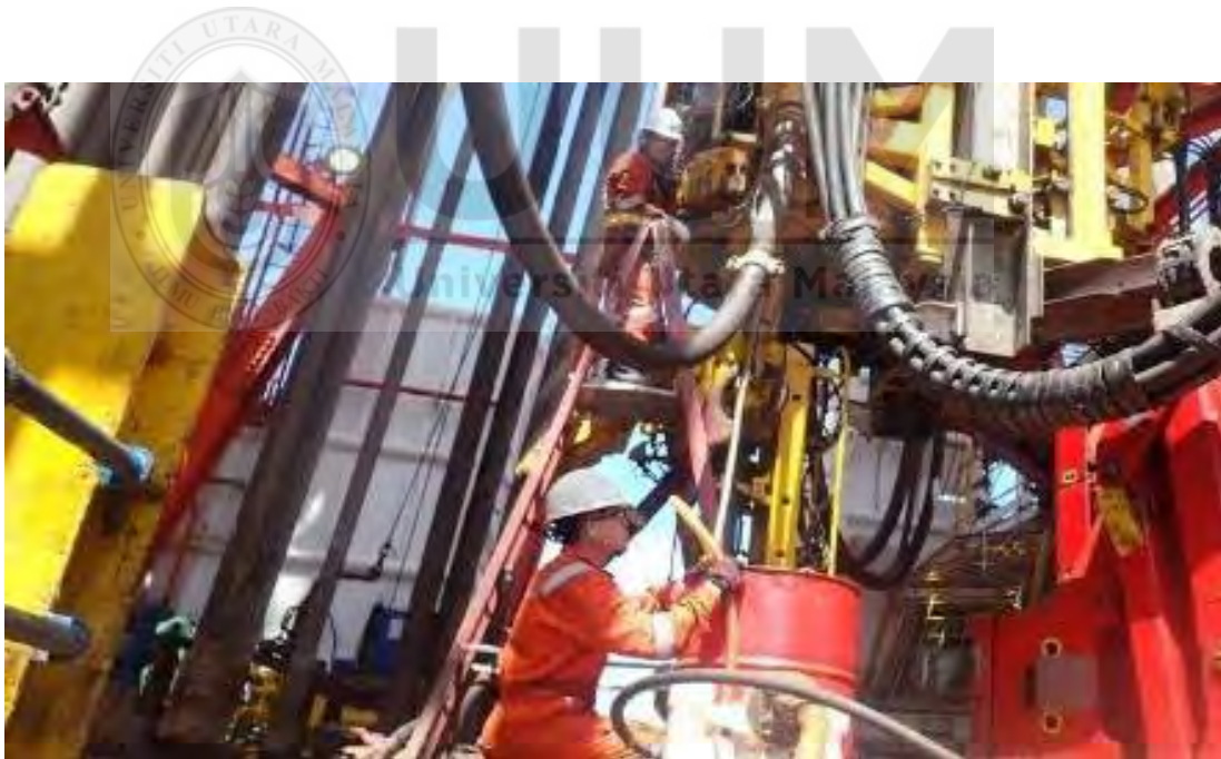
Photo 4: Observation During Power Tooling, Spot Blast - MIT & Wrapping activity [Abseiling]
