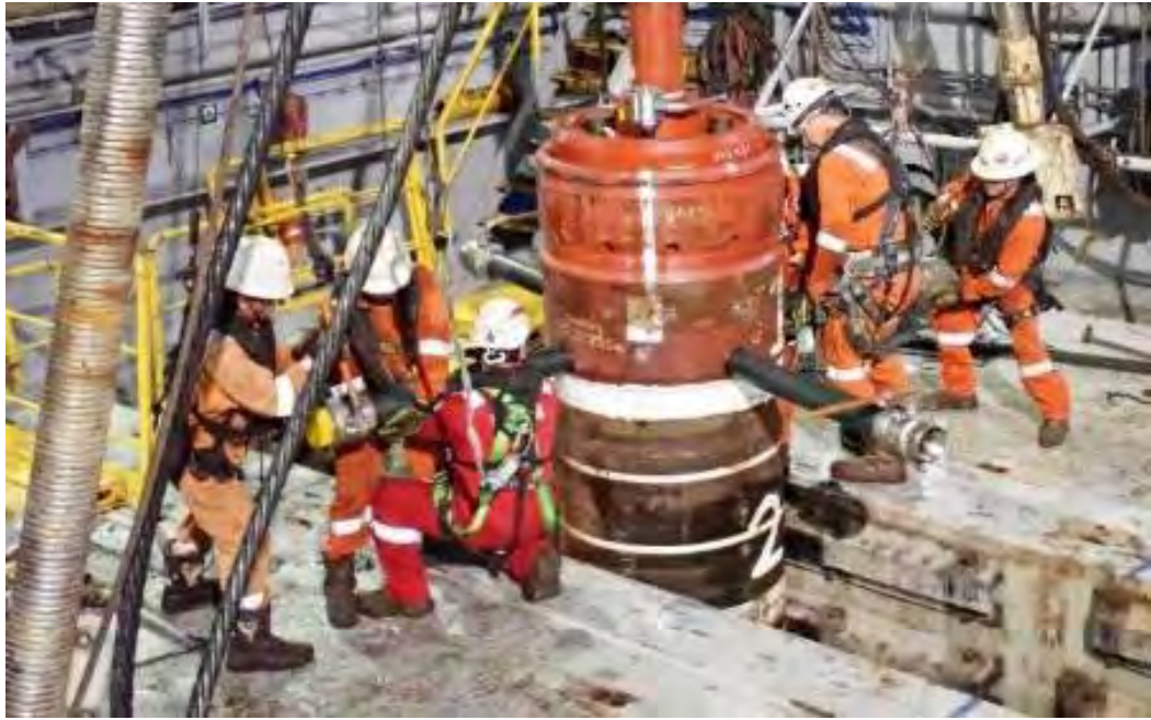
Photo 5: Observation During QC-To perform IR Gas Leak inspection on all module
