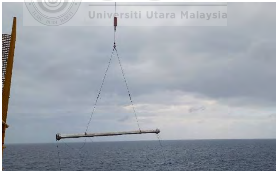
Photo 2: Observation During Routine Lifting Activity
