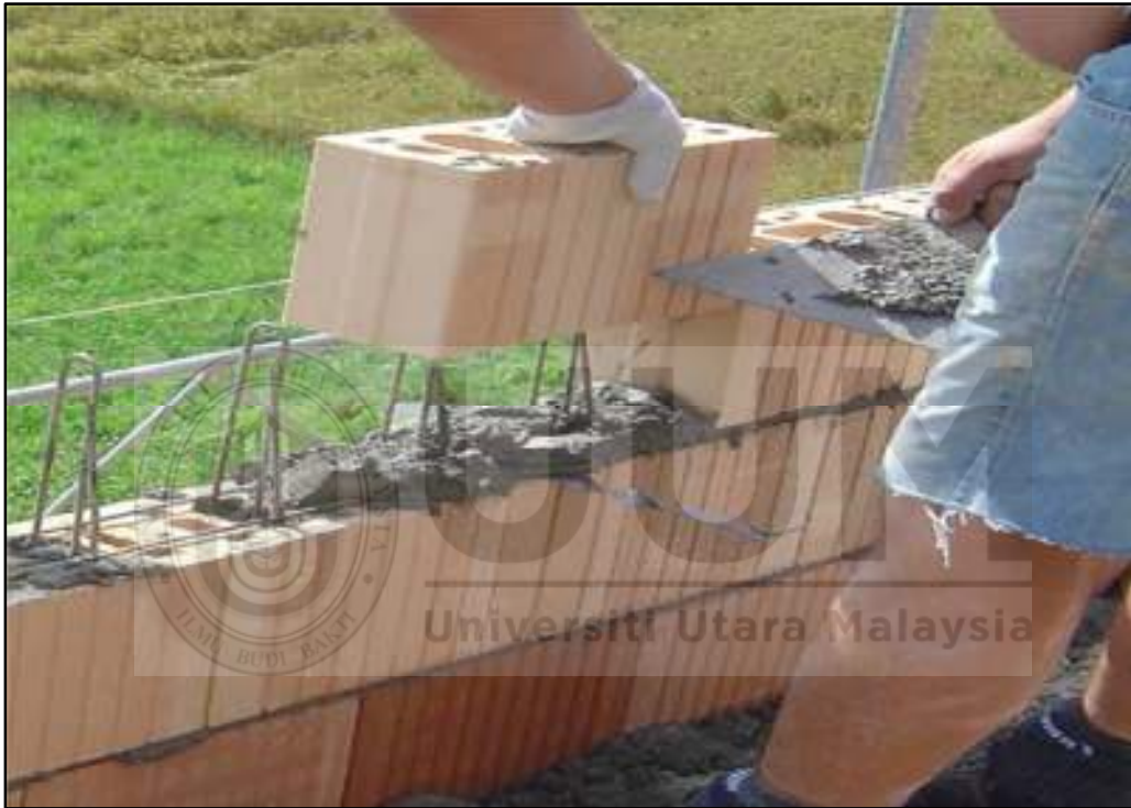
Figure 2.3 Reinforced Masonry Source: Lourence et al. (2008)
