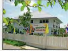
Main Building & Sign Board
